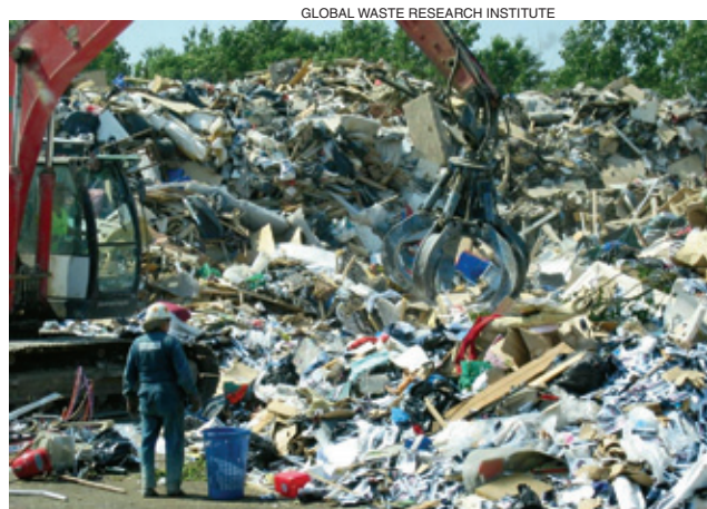
Piles of rubble from building construction and demolition sites await processing at a California recycling facility. It is feasible to regenerate that waste asphalt, concrete, and other debris into usable building materials, but far too few construction industries are doing enough of it, according to European researchers who attribute the largest share of their continent's landfill waste to the construction industry. Initiatives such as ZeroWIN hope to cut construction's waste output down to size.
